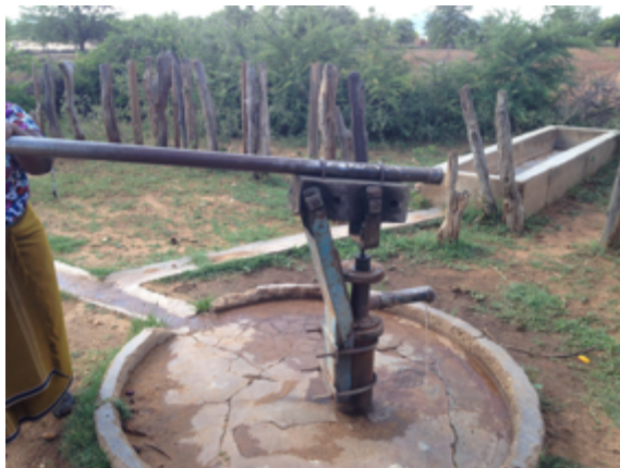
Figure 9: Chipiro borehole pump
